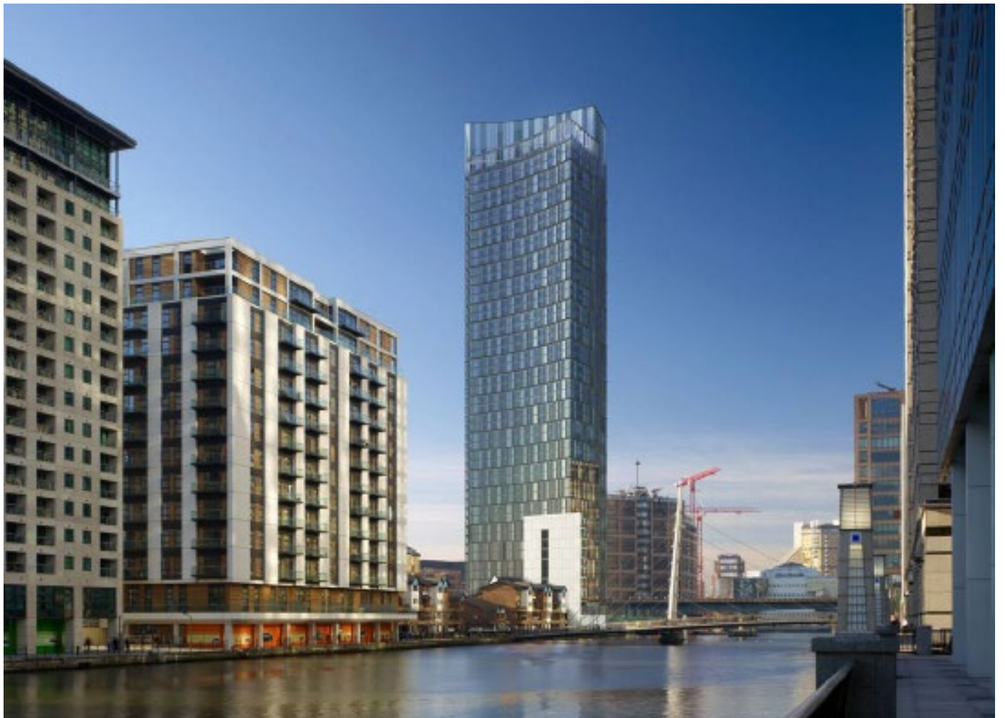
Mixed Use: South Quay- (top) CGI image From Dock side, (bottom) Axonometric of Lower Levels of Hospital Scheme
